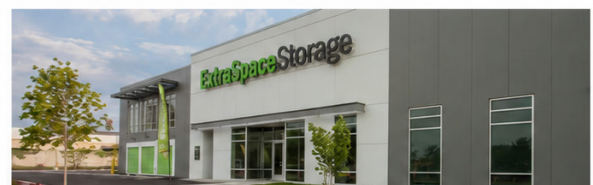
EXTRA SPACE (MANAGED) MINNEAPOLIS 86,742 NRSF | 964 UNITS
